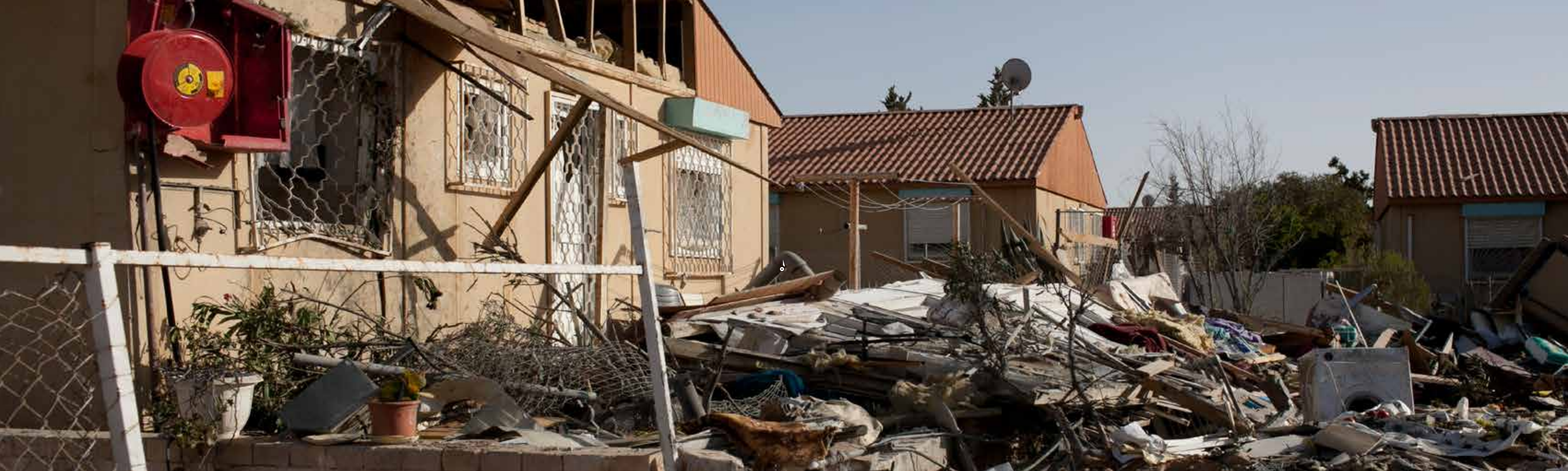
An Israeli home damaged by a rocket from Gaza.
